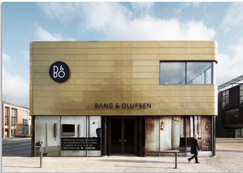
Partner owned store in Herning, Denmark
